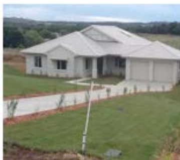
Northern side of Site - 2011 home
