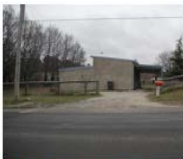
South Western side of Site - Original brick dwelling
